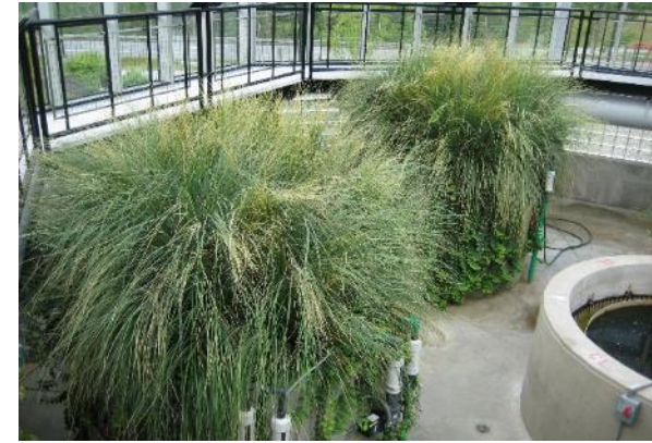
Closed Anoxic and Aerobic Reactors Filter Odors
