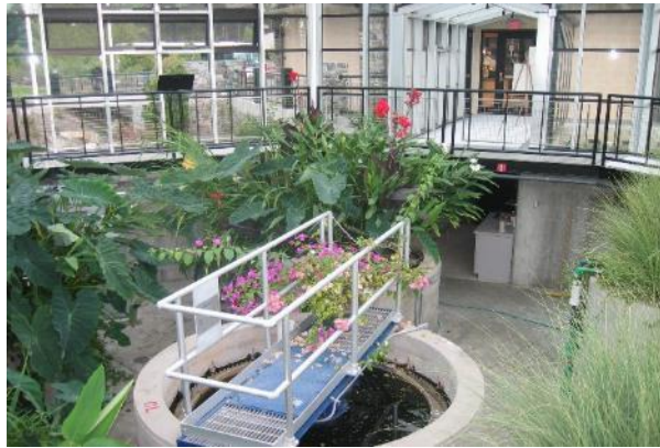
A Clarifier Settles Out Solids
